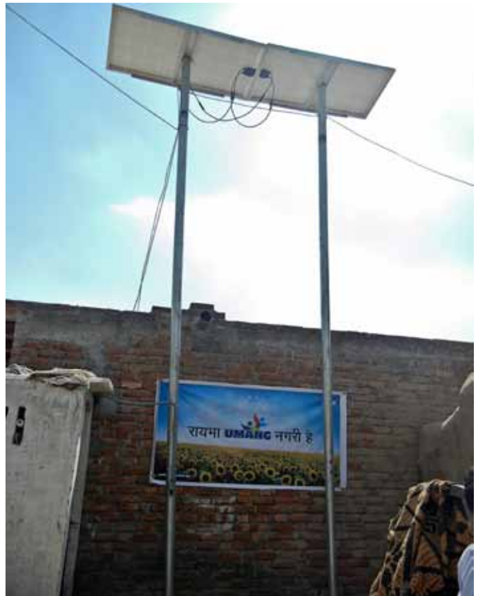
A mini powergrid enables off-grid households to have access to electricity supply.
